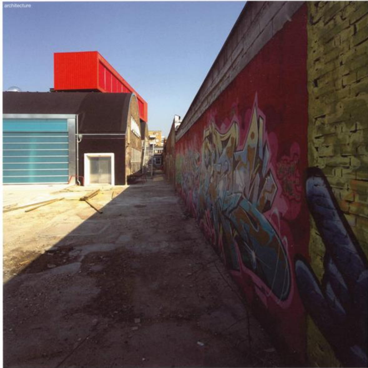
Instead of cleaning the courtyard wall of Sjakket of its graffiti, the architects integrated it into their rough-and-ready design
